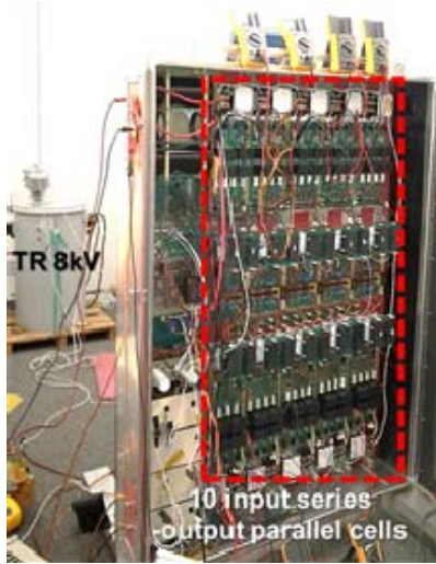
Fig. 4. Photograph of the modular multilevel front-end converter under testing.
